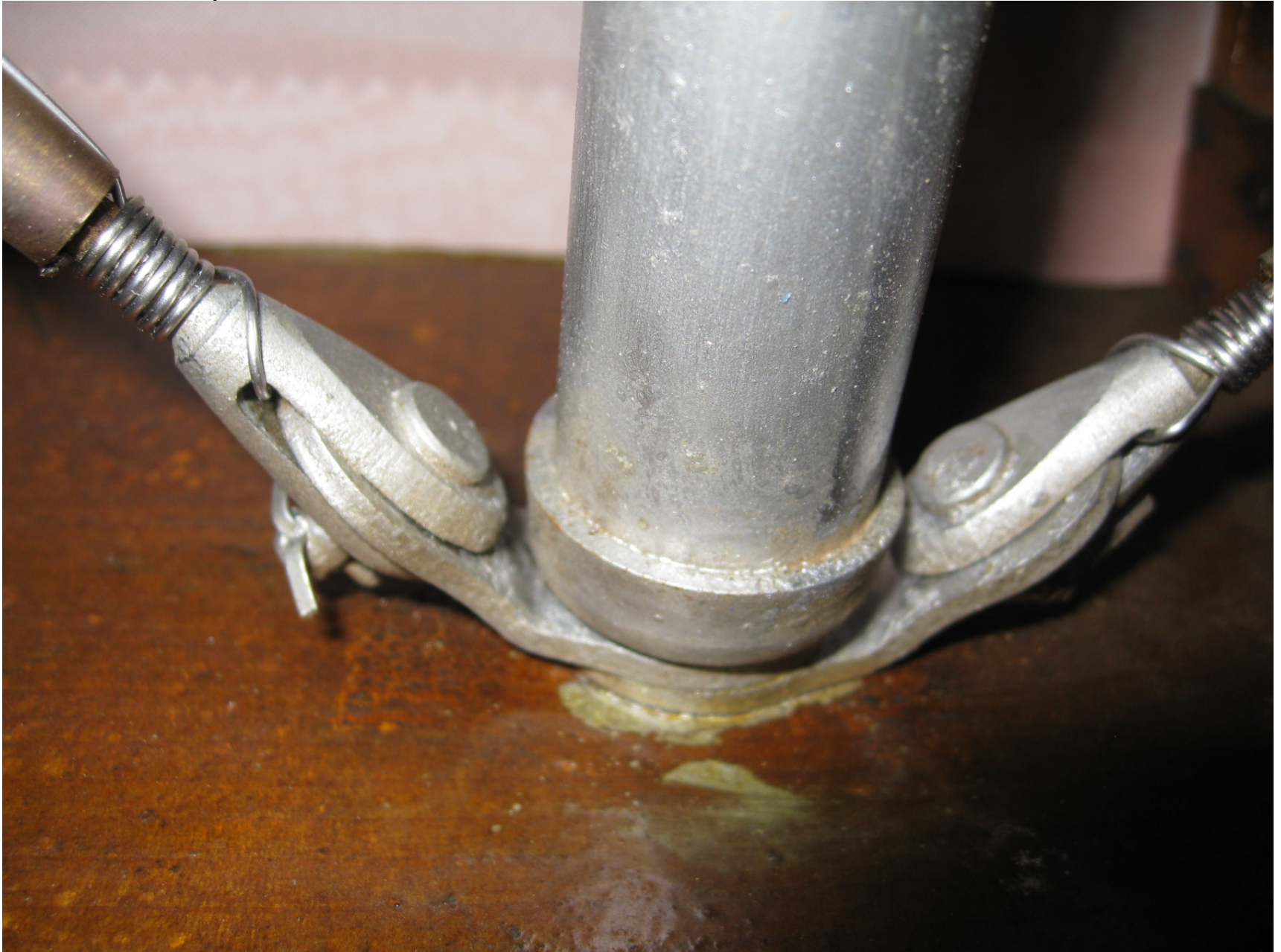
Inside Inspection Plate # 22
