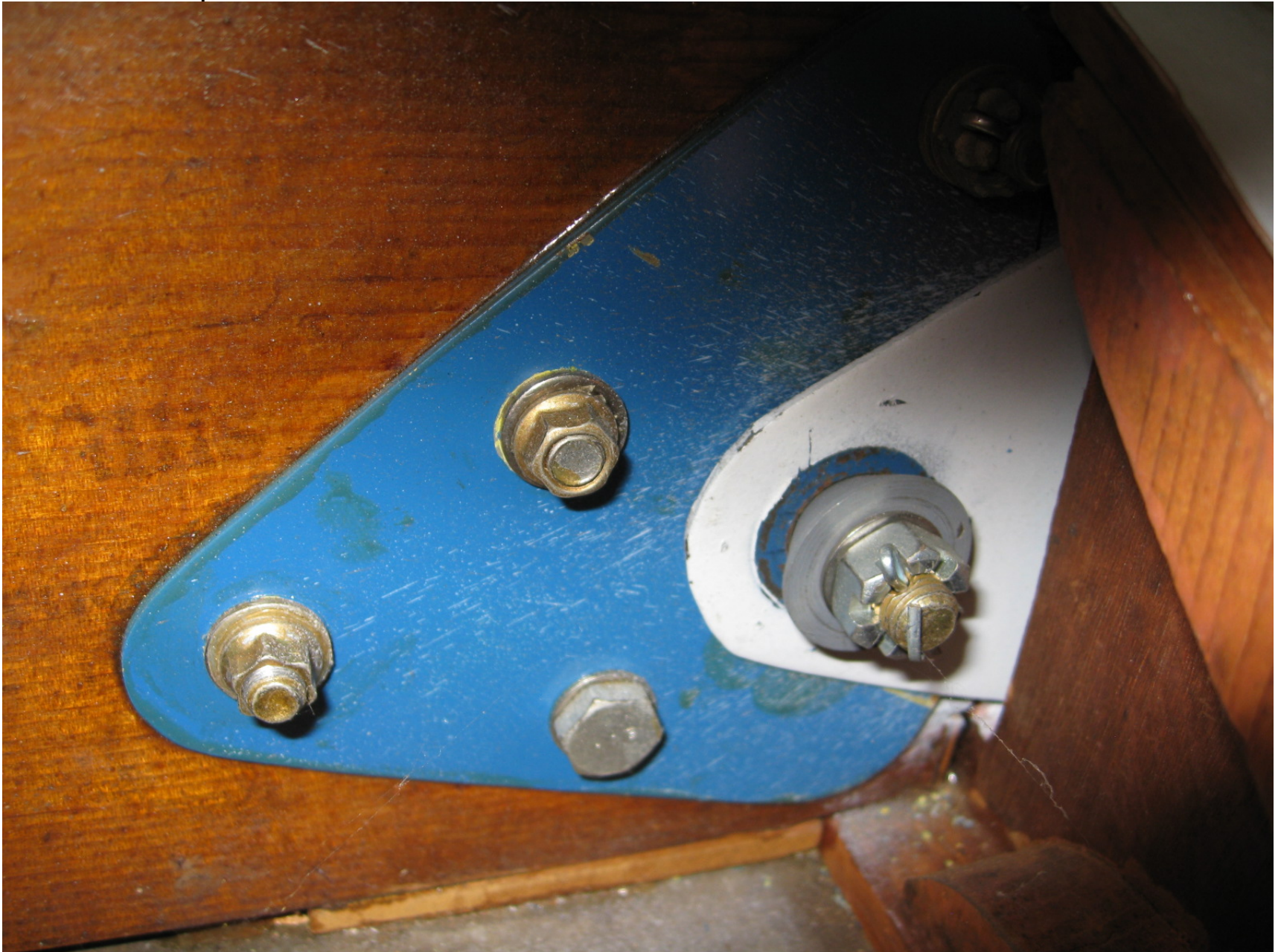
Inside Inspection Plate # 26a
