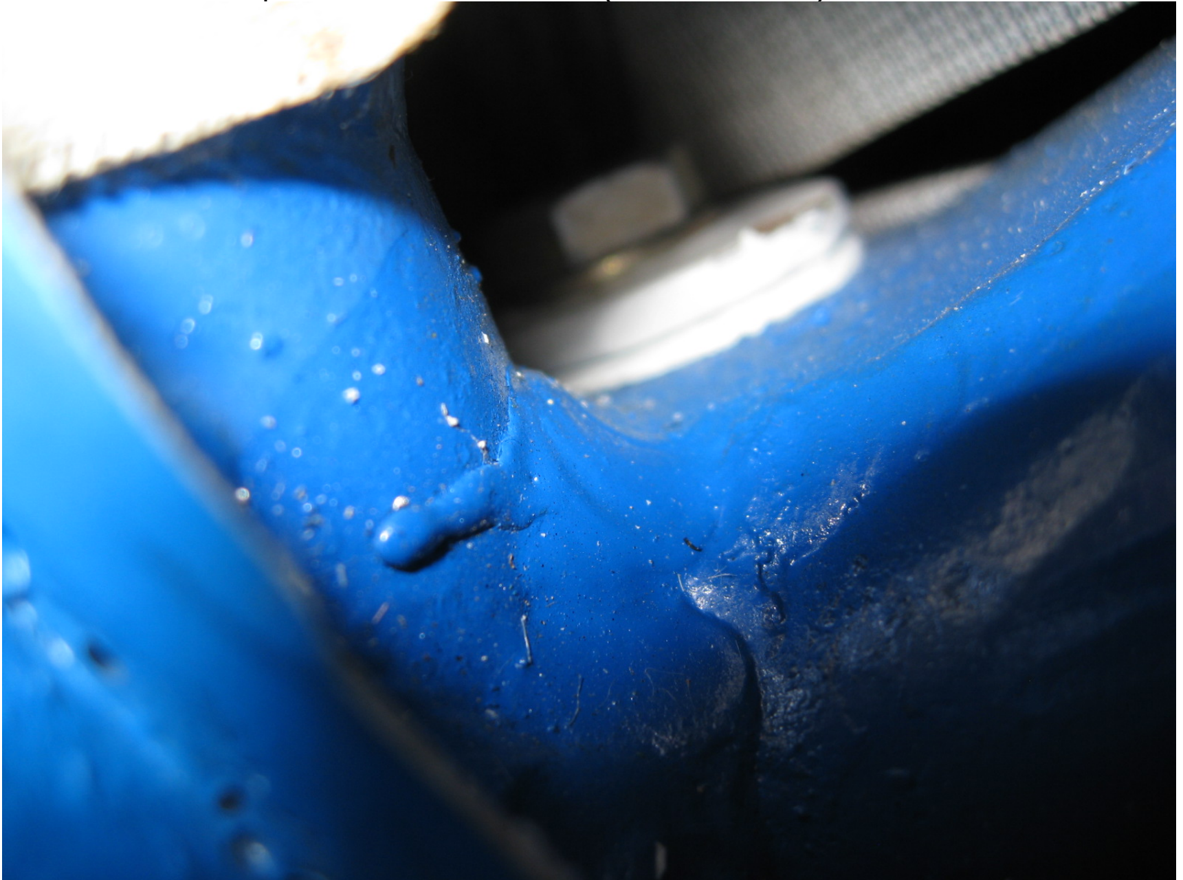
Inside Inspection Plate # 29 (#37 Similar)
