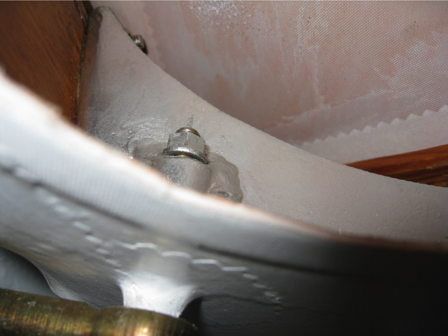
Inside Inspection Plate # 16
