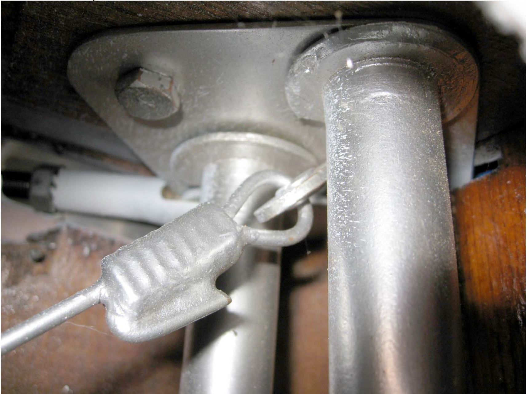
Inside Inspection Plate # 2
