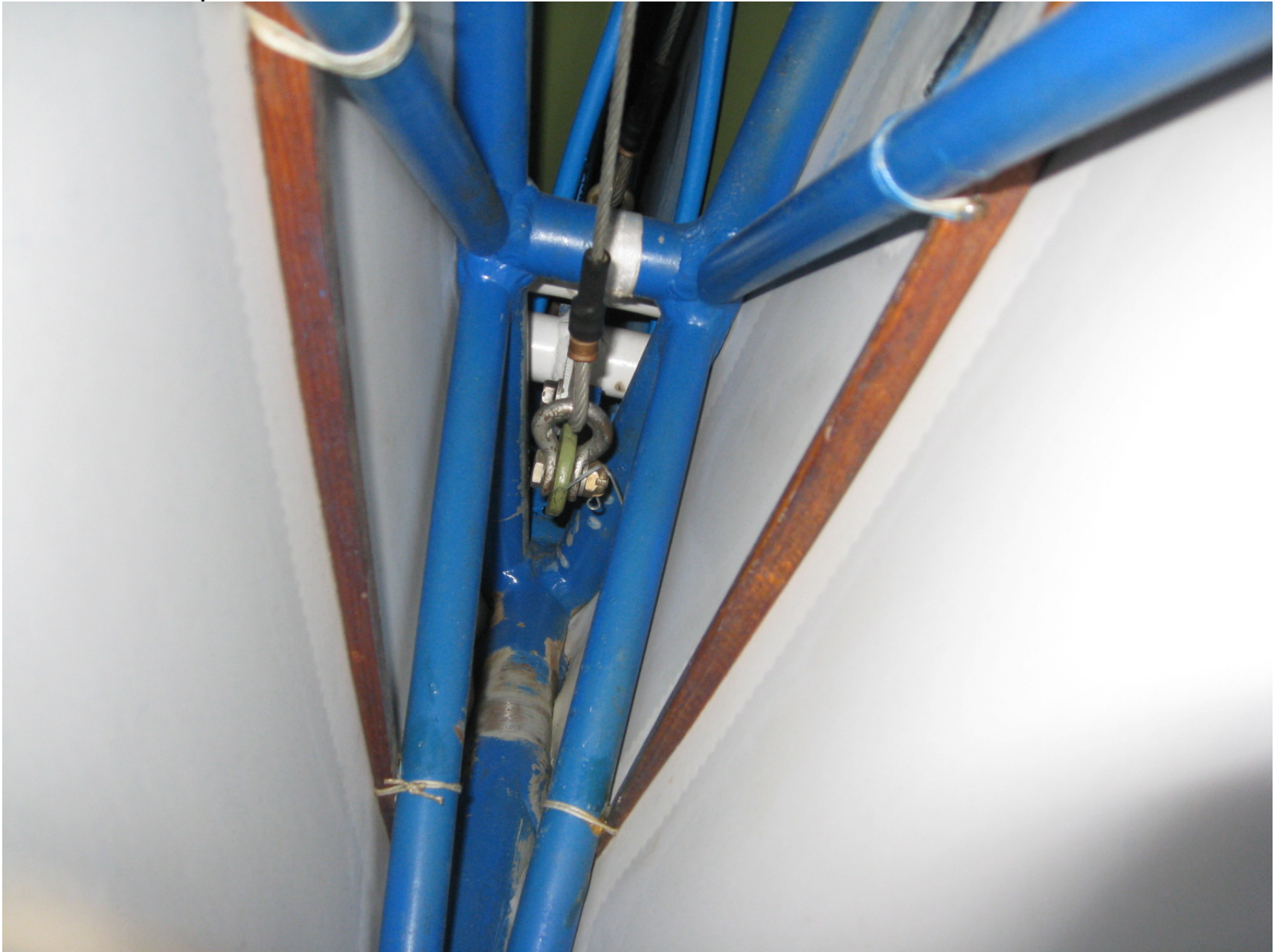
Inside Inspection Plate # 36a
