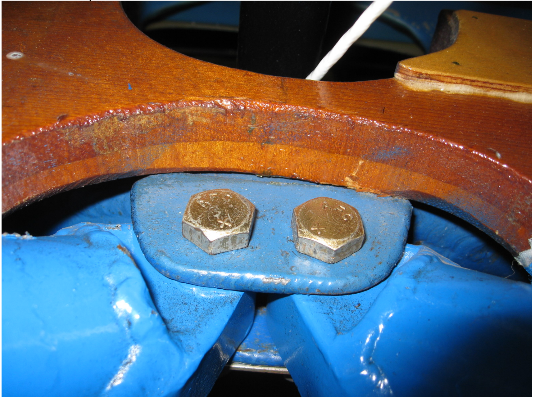
Inside Inspection Plate # 33
