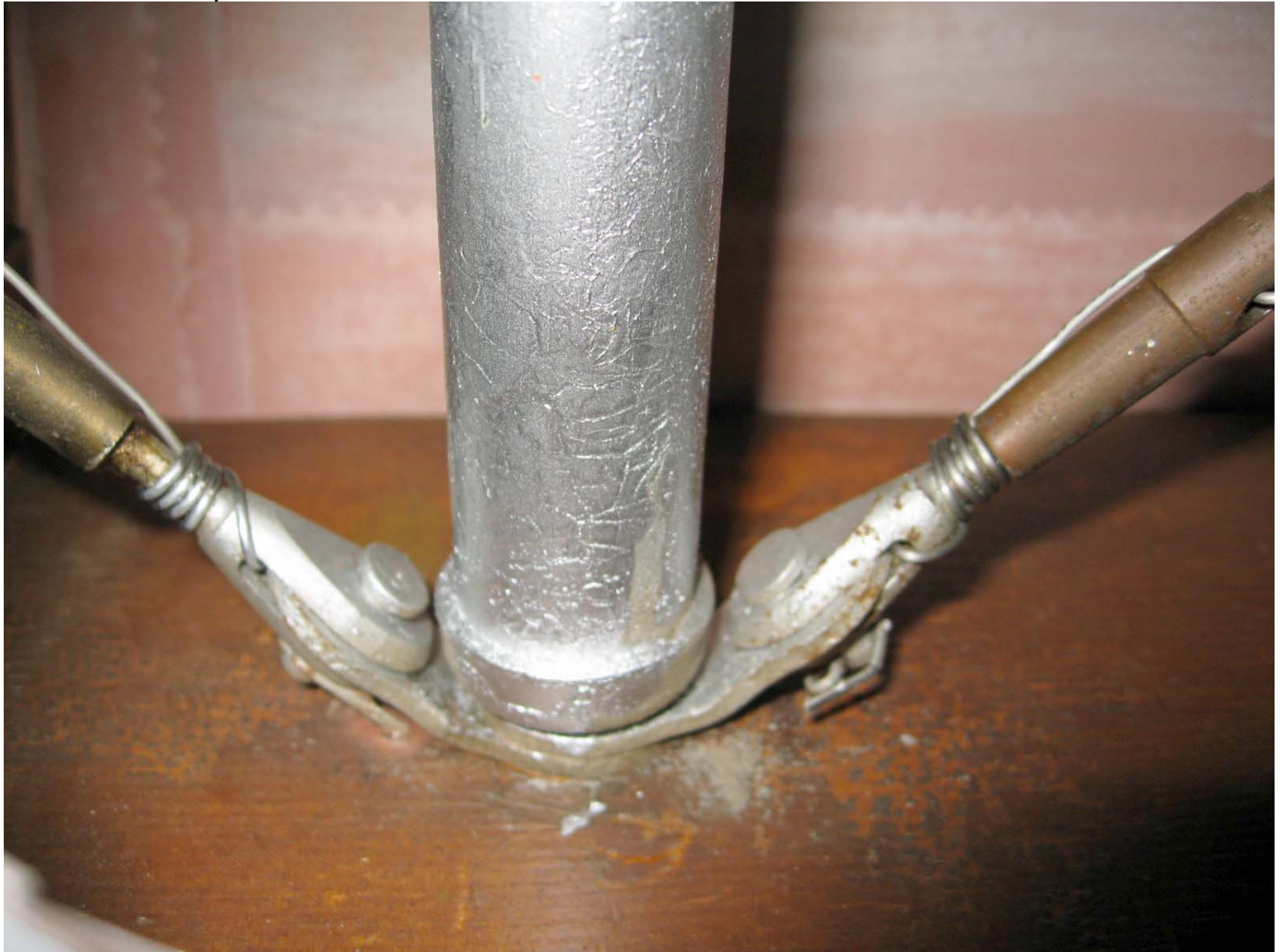
Inside Inspection Plate # 18
