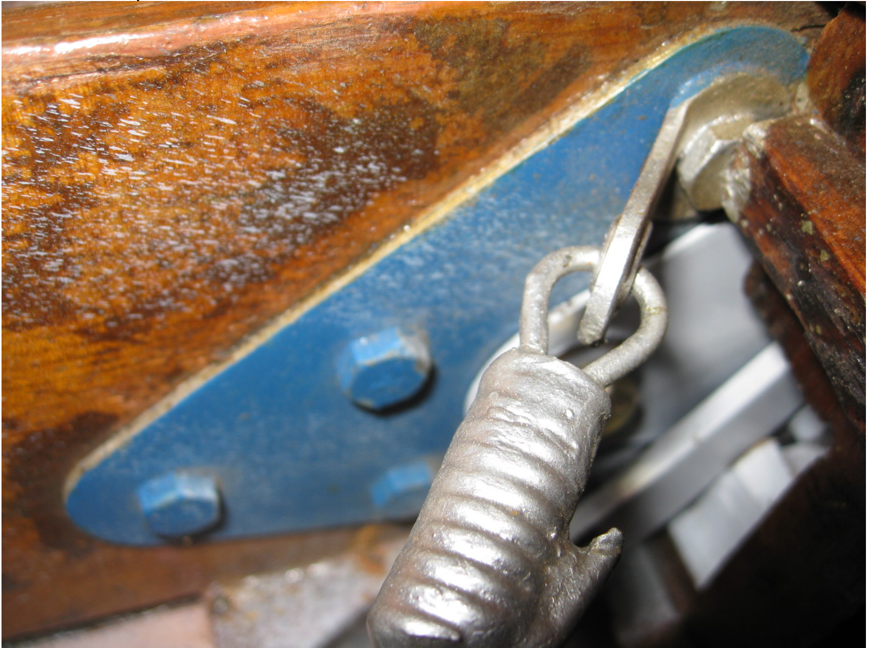
Inside Inspection Plate # 25b
