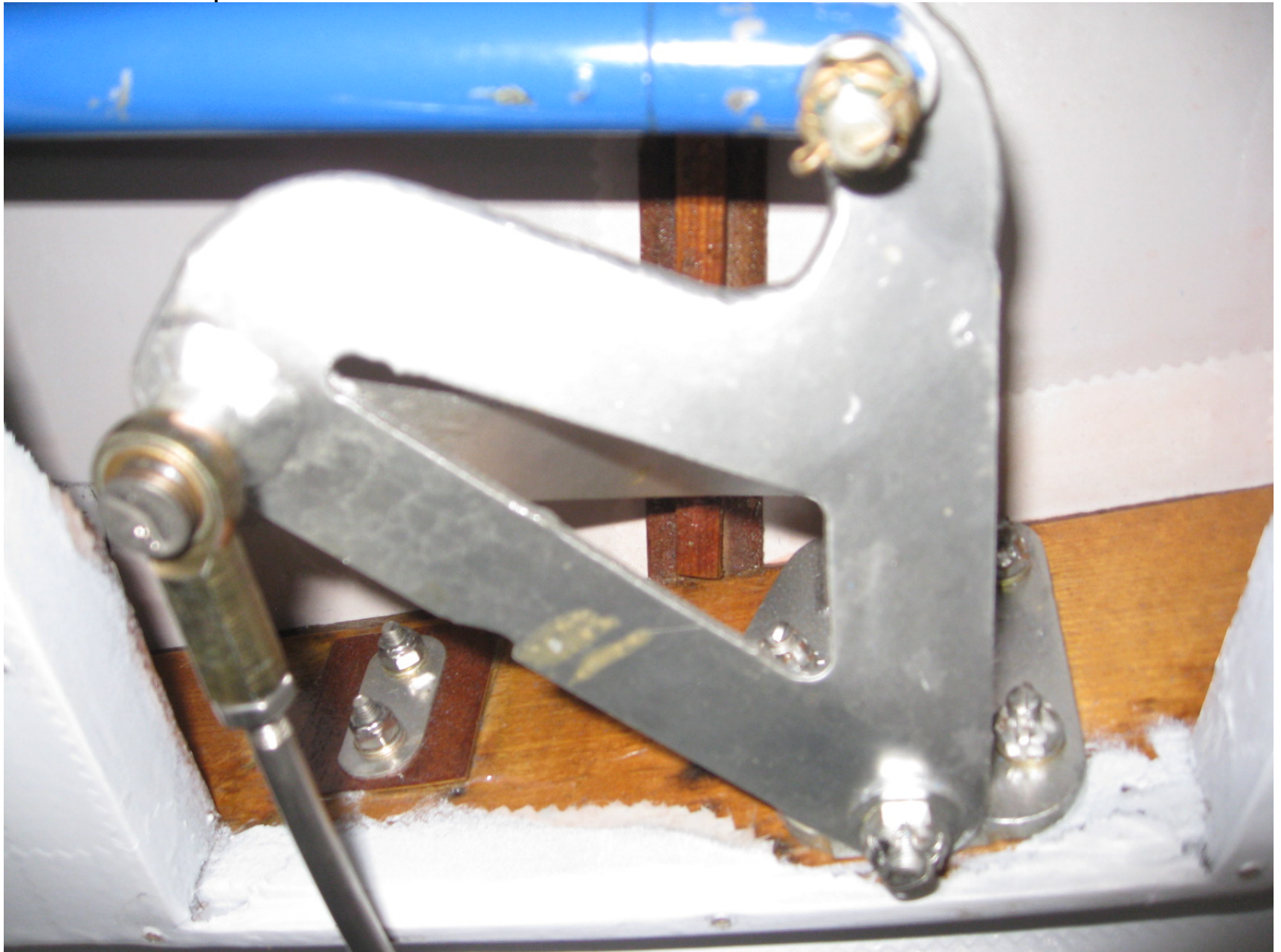
Inside Inspection Plate # 15
