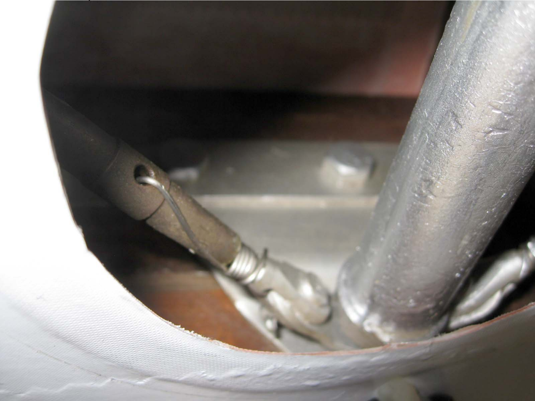
Inside Inspection Plate # 20
