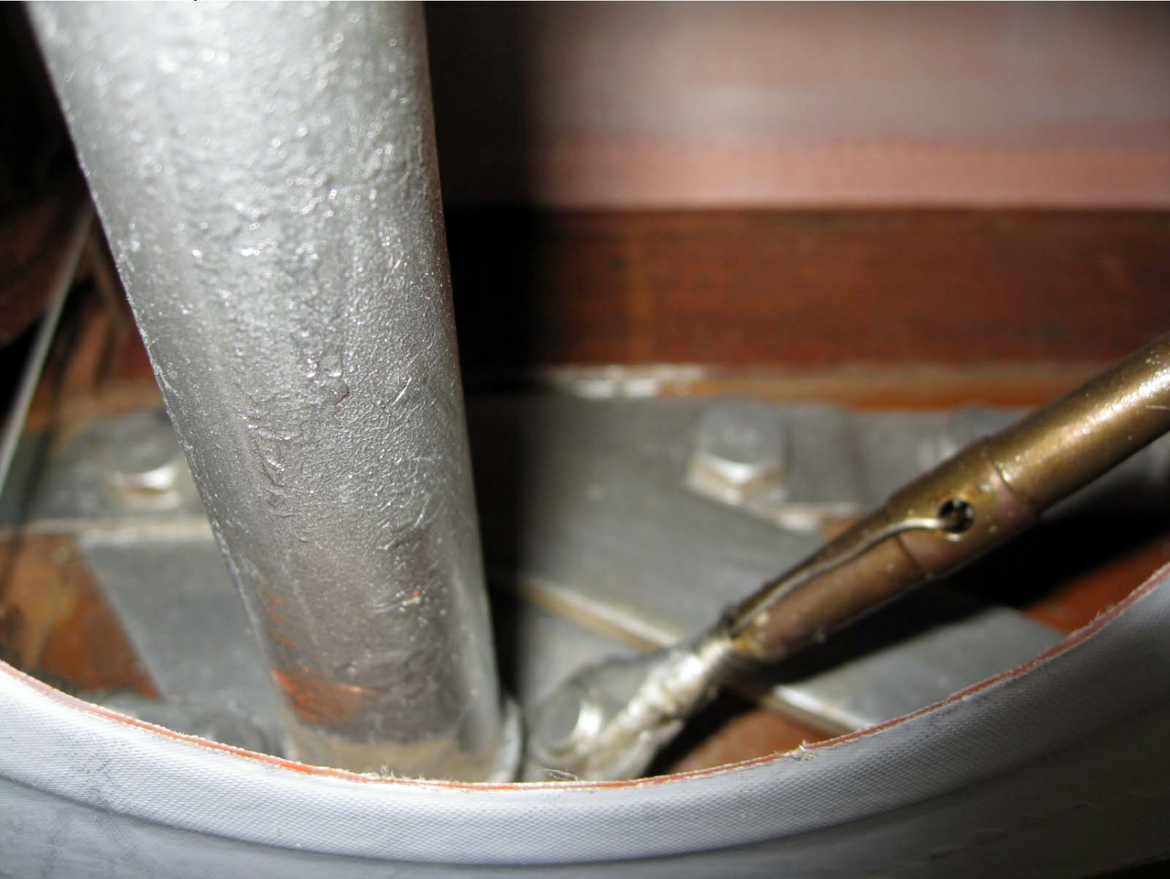
Inside Inspection Plate # 19
