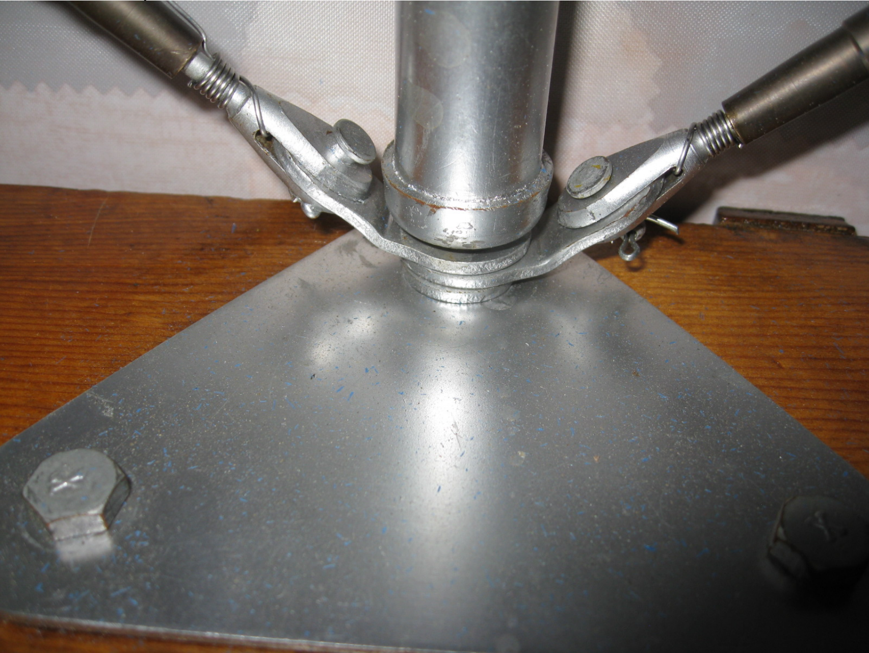
Inside Inspection Plate # 14
