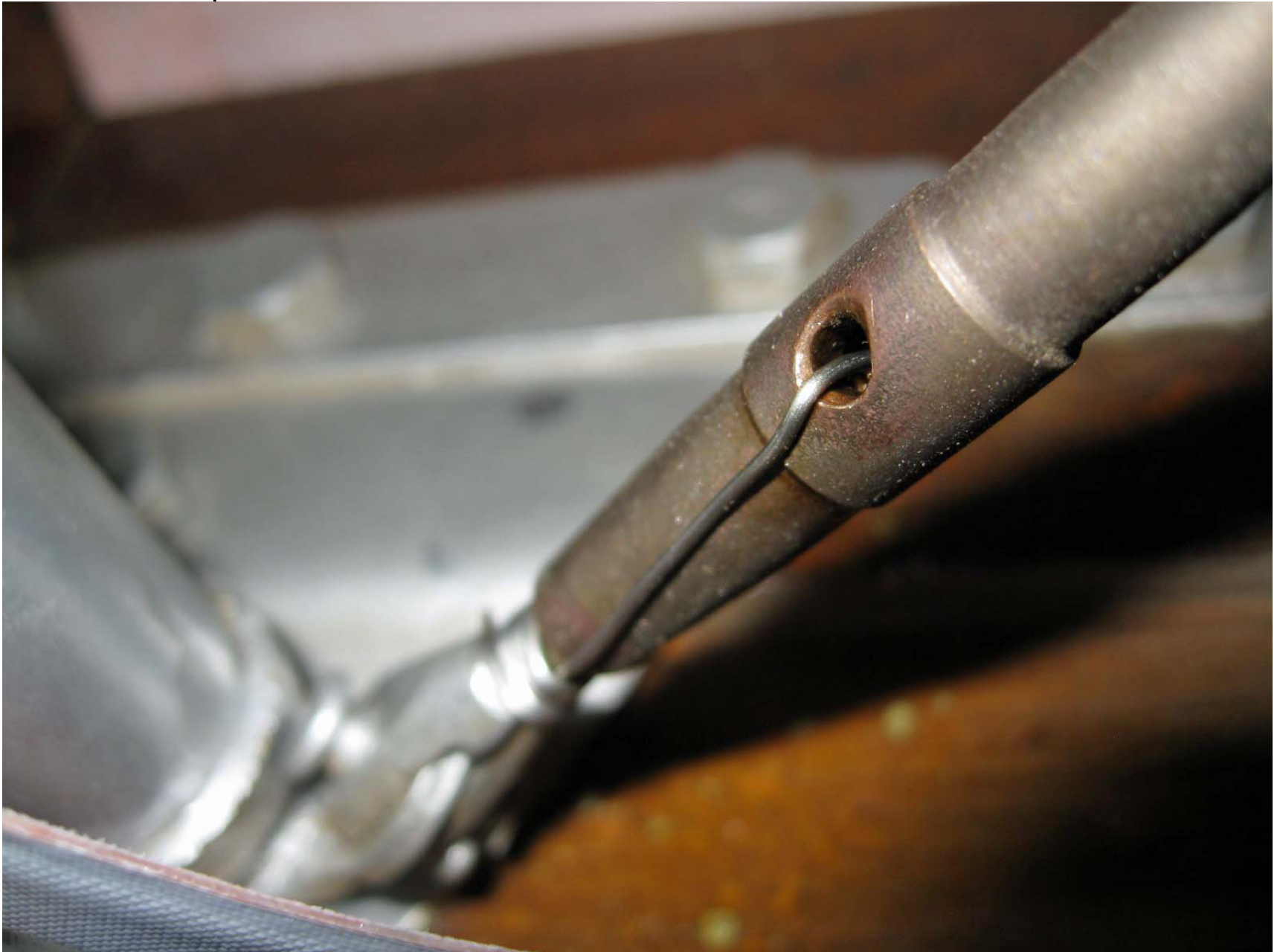
Inside Inspection Plate # 24
