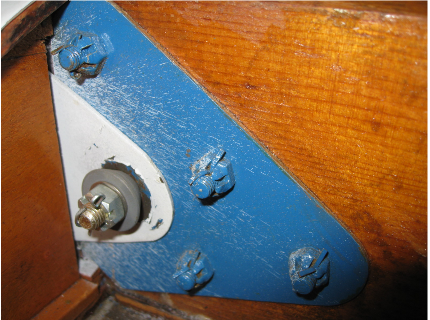
Inside Inspection Plate # 25a
