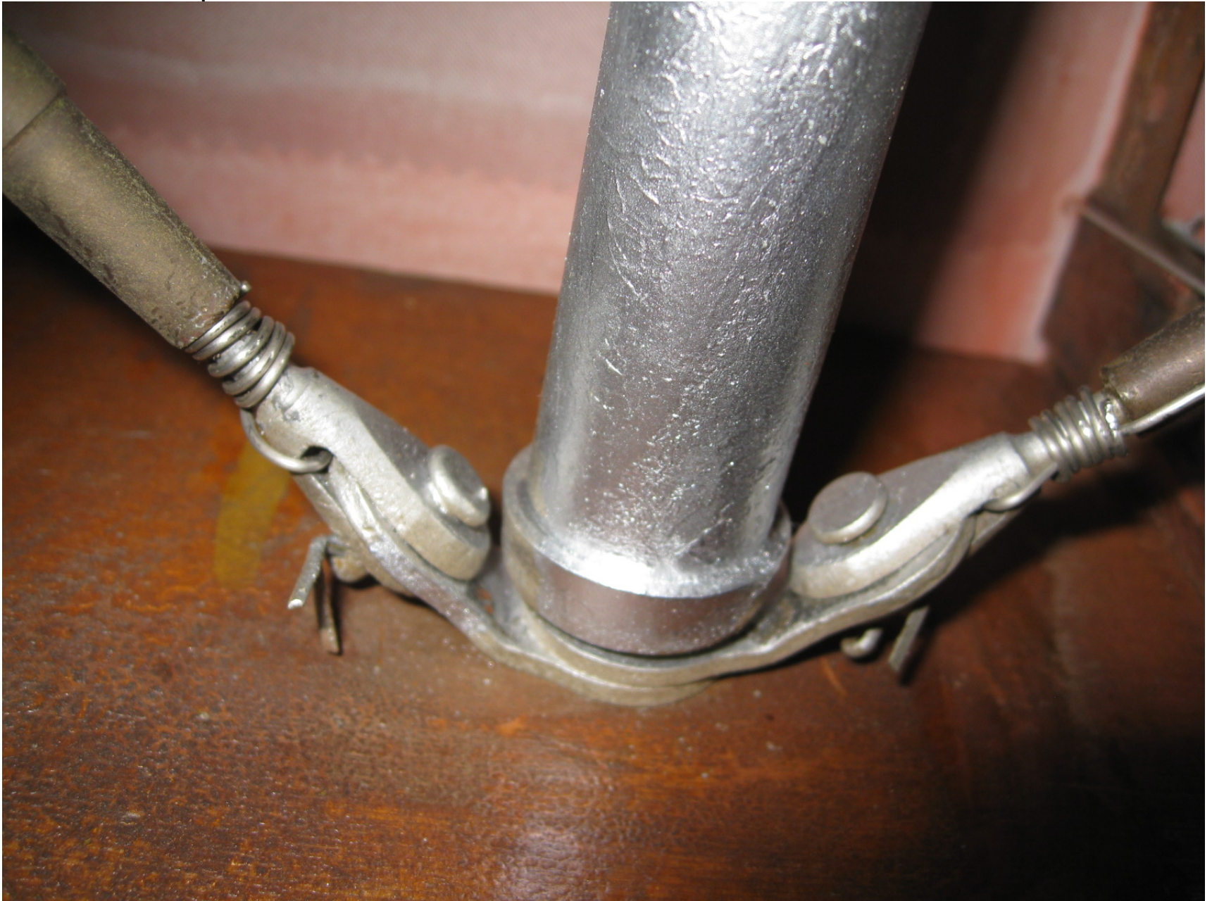
Inside Inspection Plate # 17
