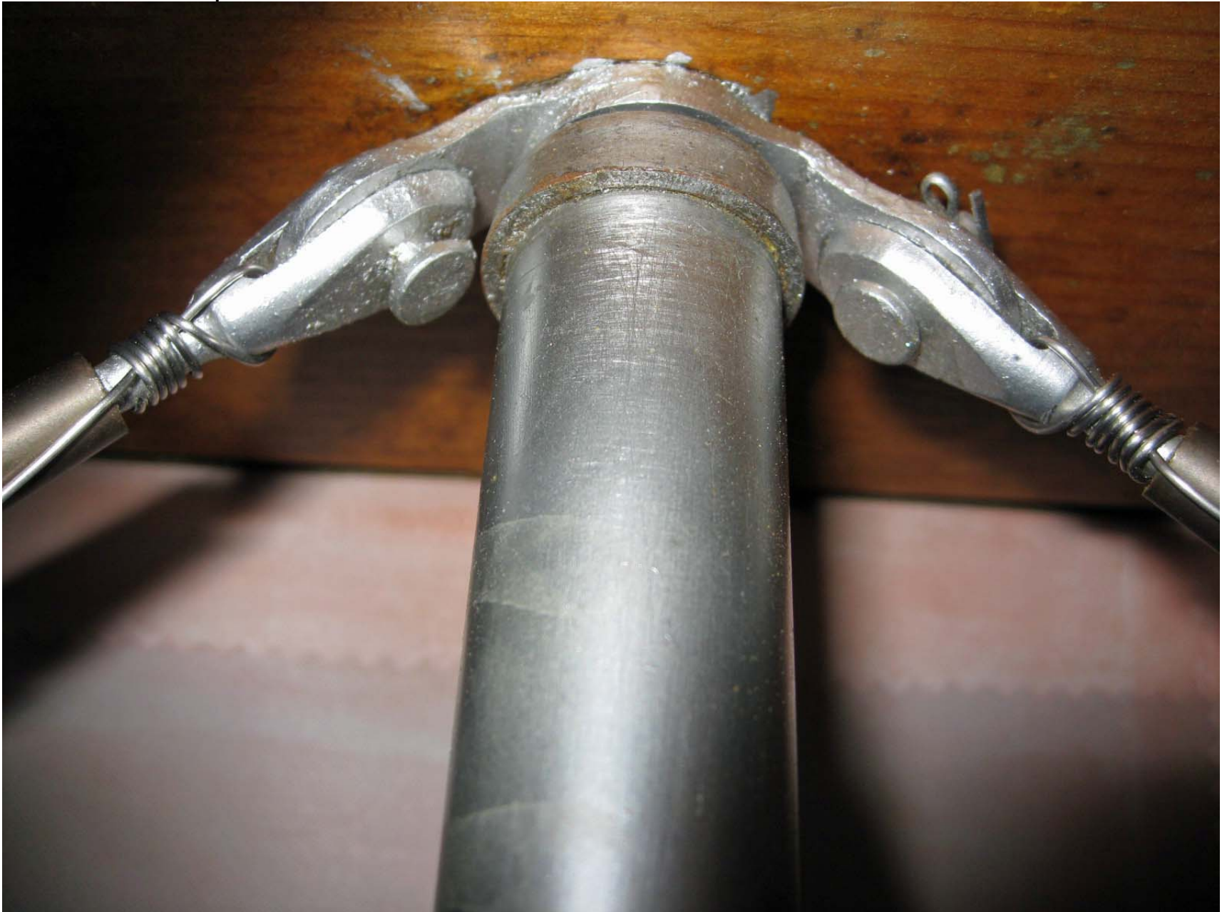
Inside Inspection Plate # 3
