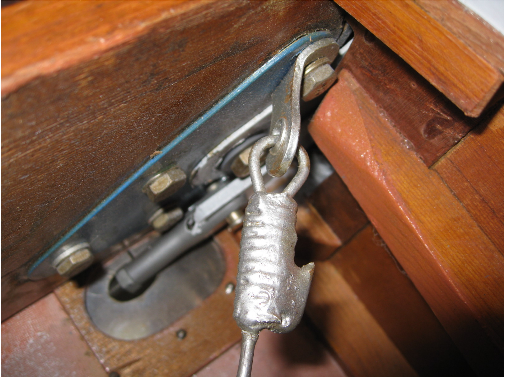
Inside Inspection Plate # 28a
