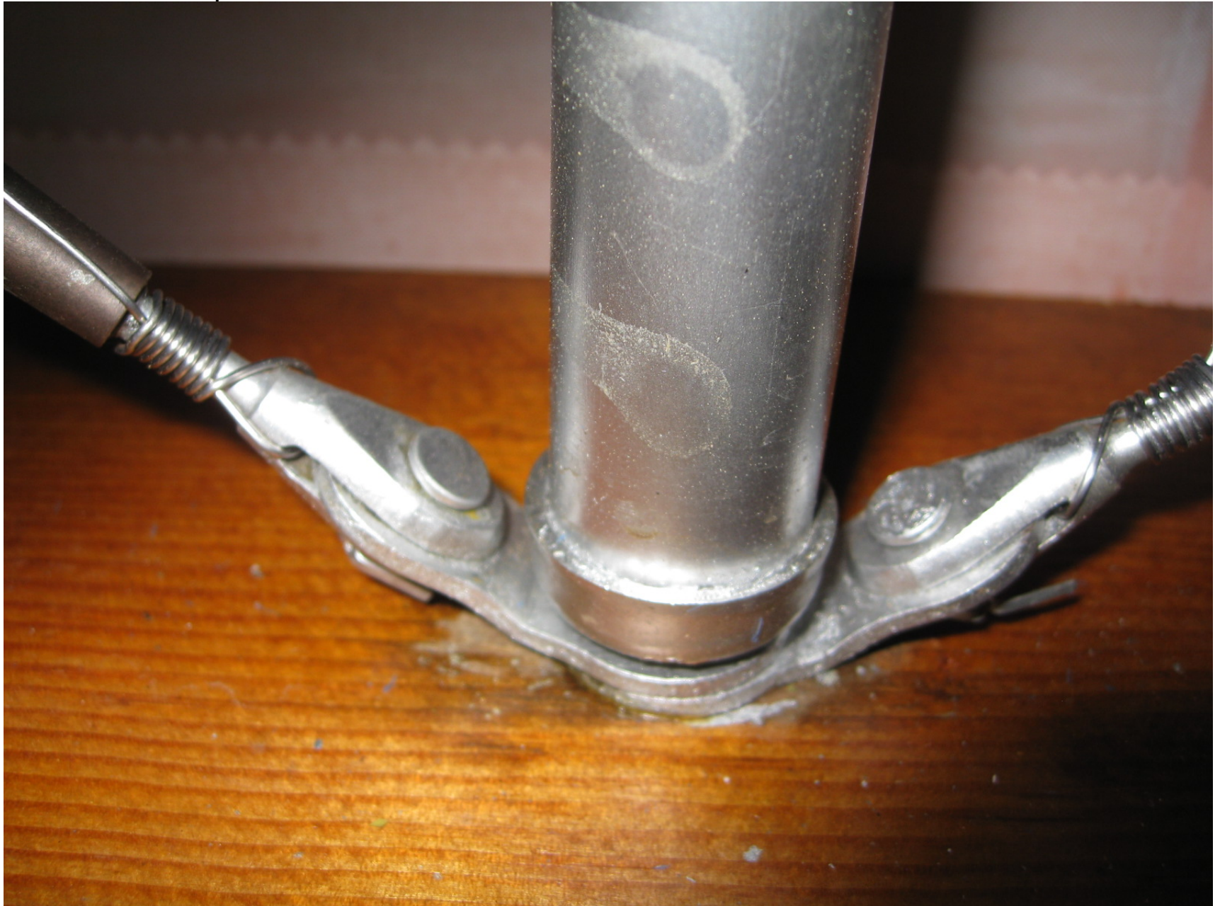
Inside Inspection Plate # 4
