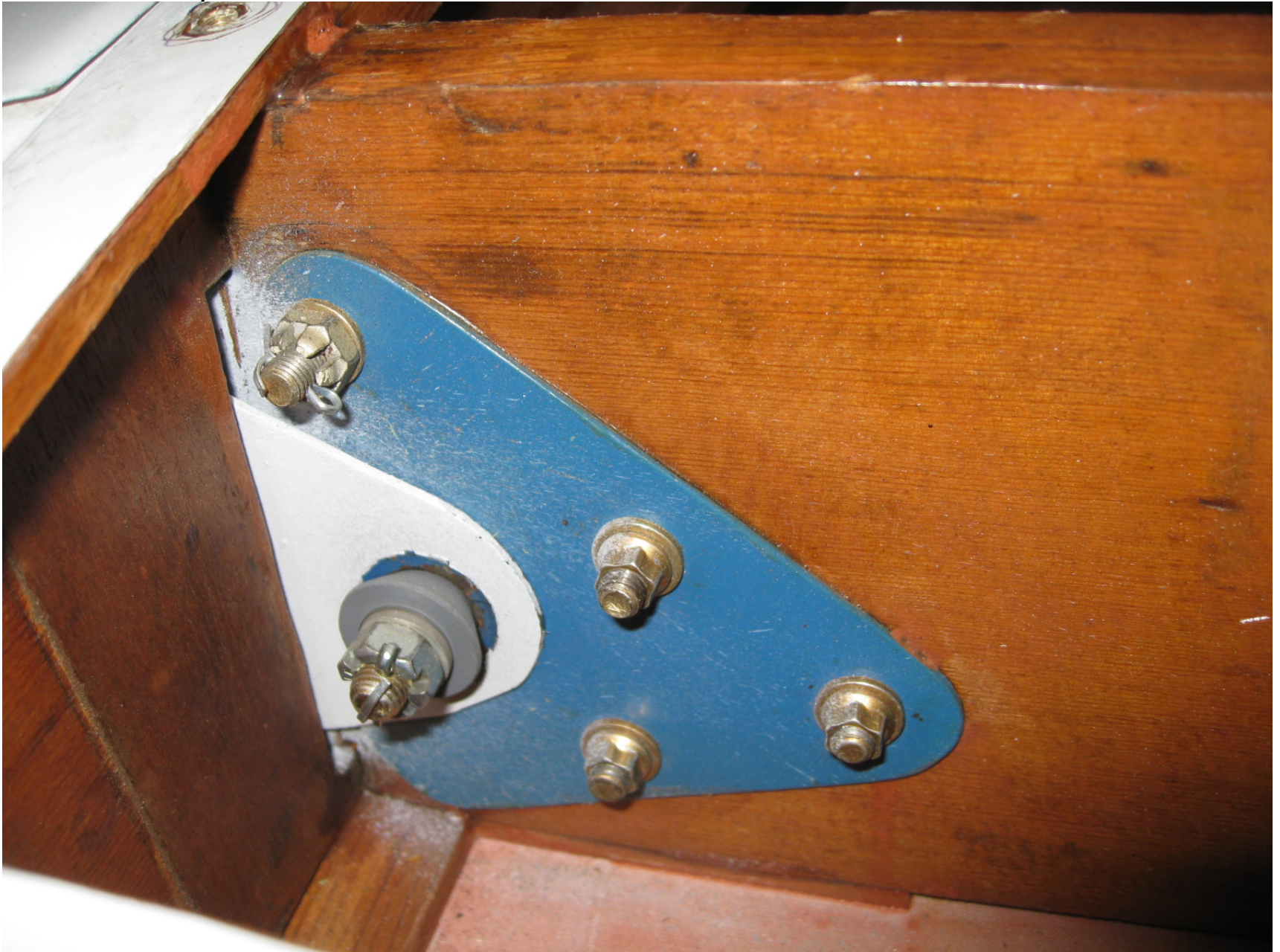
Inside Inspection Plate # 28b
